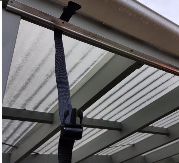
**4** Slide the blind into the rope track. You can now continue with the installation, as per the Zip or Tension Patio Blind Installation Instructions.
