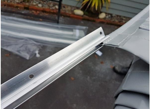
**4A** Slide the stowage straps into position, behind the second hole in from each side. Ensure the female end of the strap is on the outside, as shown. Only the double thickness portion of the webbing should be exposed to the outside. Once in position, insert the remaining screws (gently, to avoid damaging the webbing). You can now continue with the installation, as per the Zip or Tension Patio Blind Installation Instructions.
