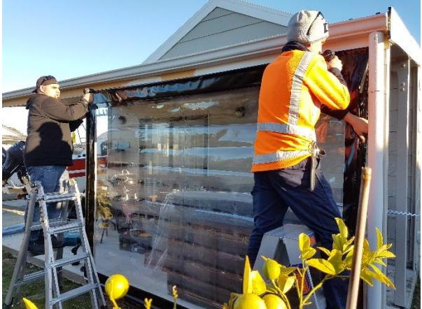
**5** Insert the stowage straps on the top edges, as shown. The outside edges of the straps should align with the join between the Clear PVC and the border PVC.
